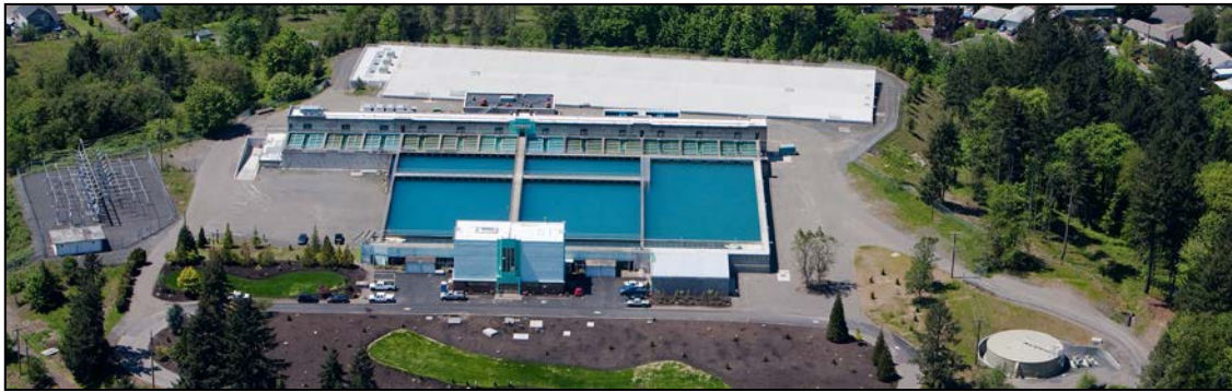
Hayden Bridge Water Treatment Plant
