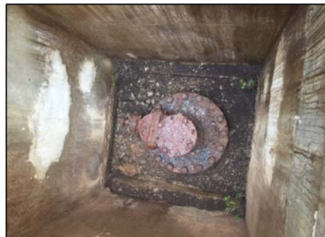
30-inch – Extract Location
